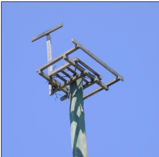
Osprey nesting platform – This design has since been revised to remove the vertical perch as crows were found to use the roost to harass the osprey for food, EPA 2000.
