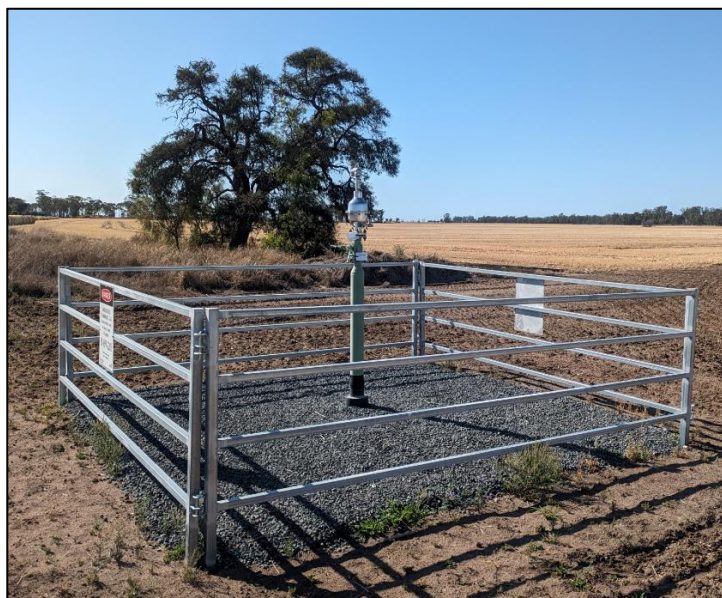
Figure 4-9 High point vent (HPV)
